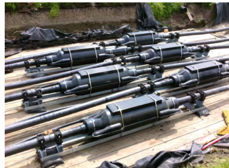
Crossbonding joints / Crossbondingmuffen
